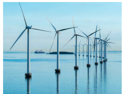
Sensors make windfarms more efficient
