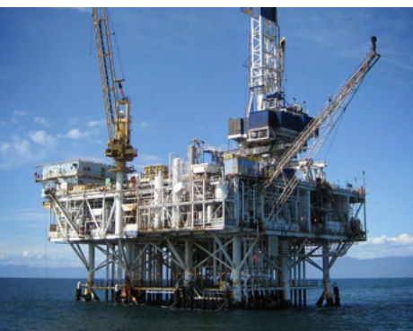
Sensors make oil & gas rigs safer
