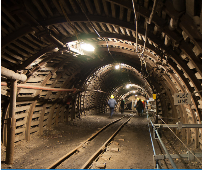
Structural Health Monitoring
